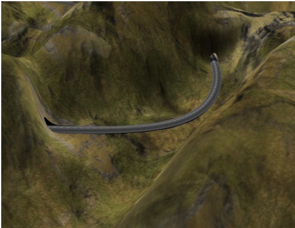
Tunnel and level Area View
